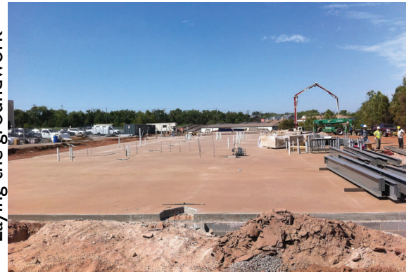
Stage One: Laying the groundwork
