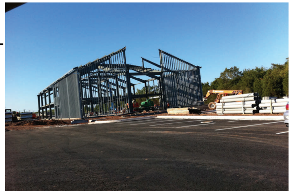
Stage Two: The structure is up.
